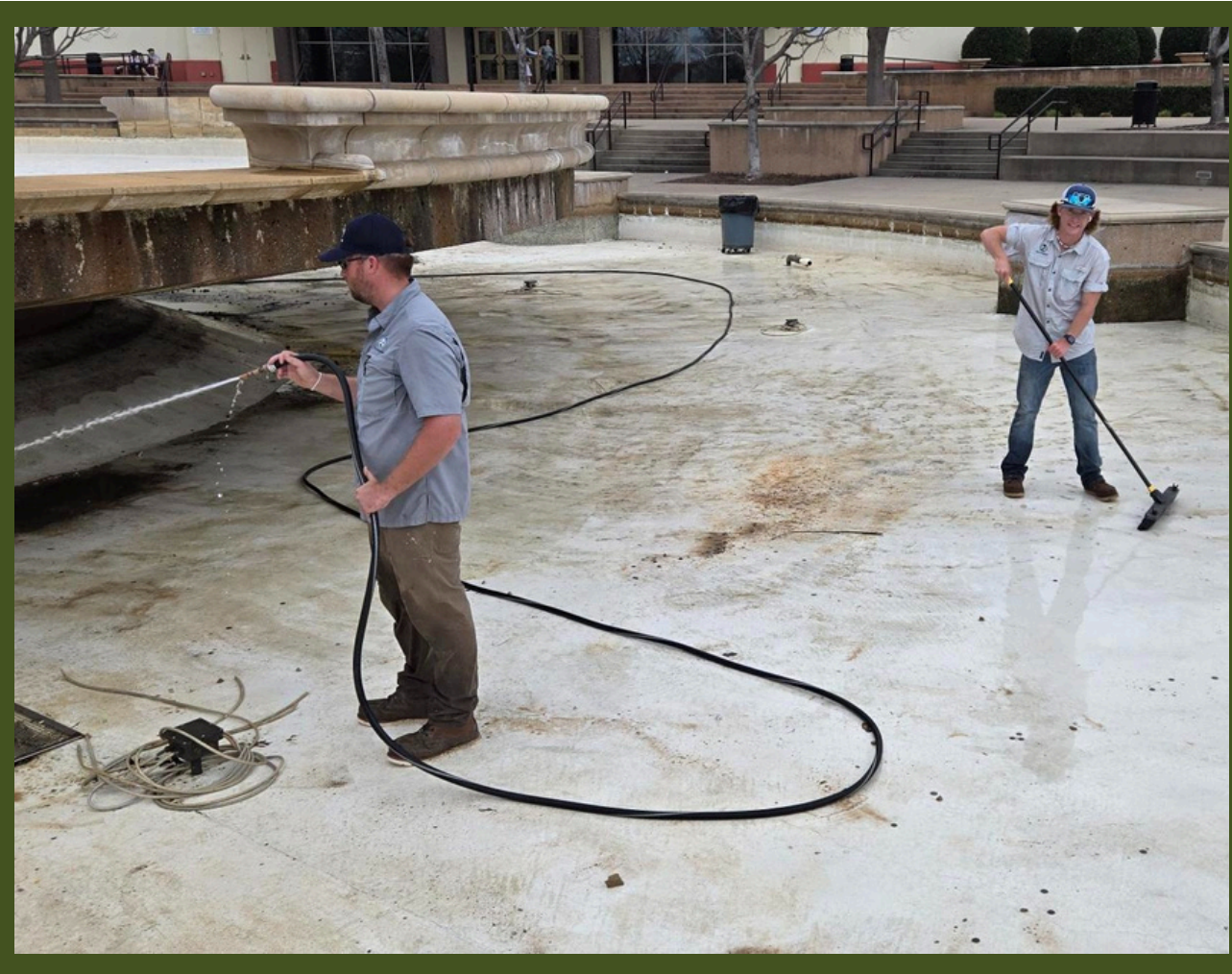
HARBOR FOUNTAIN CLEANING AND LED LIGHTING PROJECT
